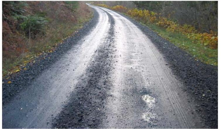
**Photo 1a & b.** Two roads in the Oregon Coast Range that had been surfaced with rock and gravel about 3 months prior to the time of photos. The travelways had primarily reverted to a native surface condition that is actively eroding, including that in concentrated runoff in ruts in the native surface of the roads, resulting in high levels of sediment delivered to nearby streams.
